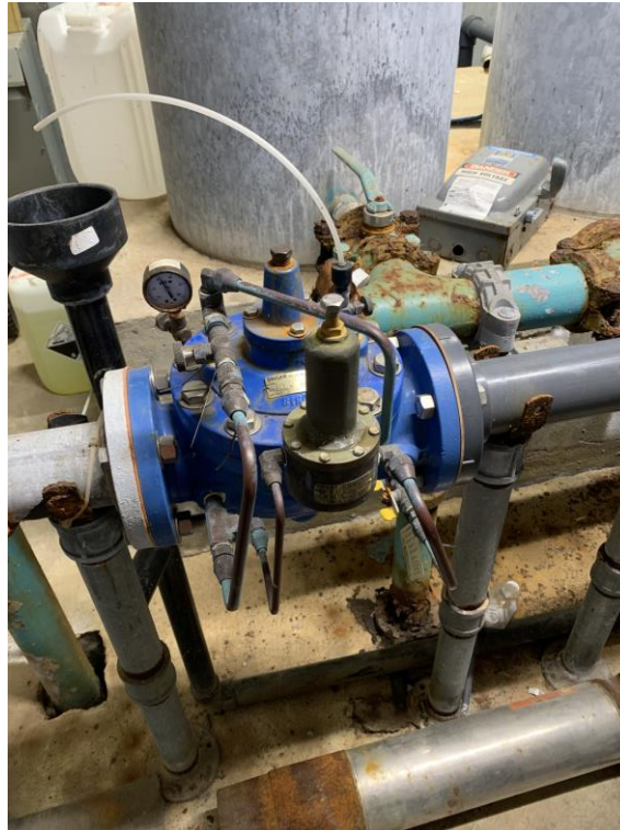
Figure A.8: Isolation Ball Valve Downstream of Flow Control Valve
