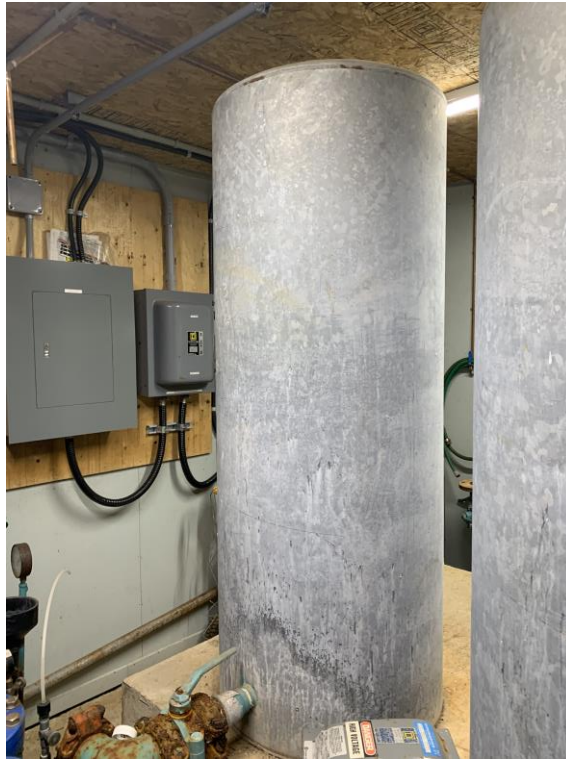
Figure A.14: Northwest Pressure Tank Butterfly Isolation Valve. The Valve is Significantly Corroded but Still Operational
