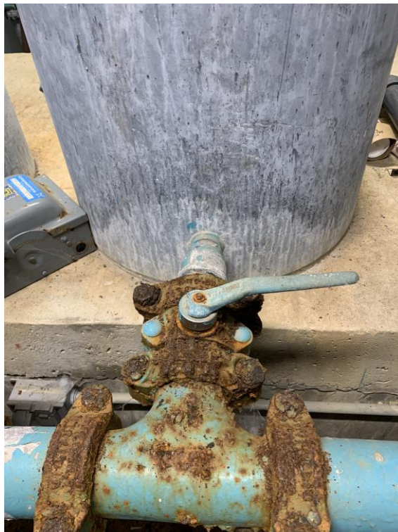
Figure A.16: Southwest Pressure Tank Butterfly Isolation Valve. The Valve is Significantly Corroded but Still Operational
