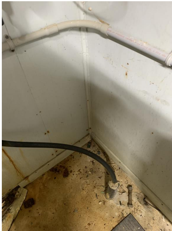
Figure A.22: Water Service Line Floor Penetration
