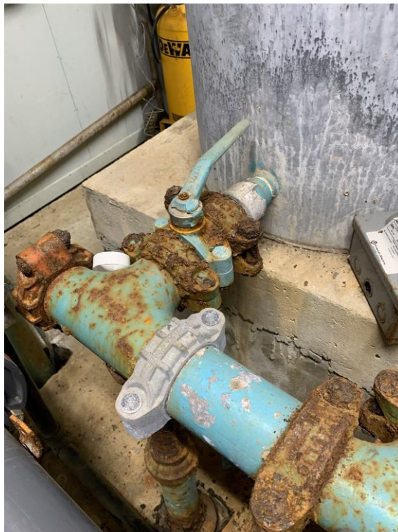
Figure A.14: Northwest Pressure Tank Butterfly Isolation Valve. The Valve is Significantly Corroded but Still Operational
