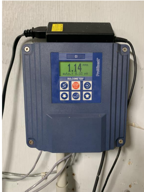
Figure A.25: Free Chlorine and pH Analyzer Display
