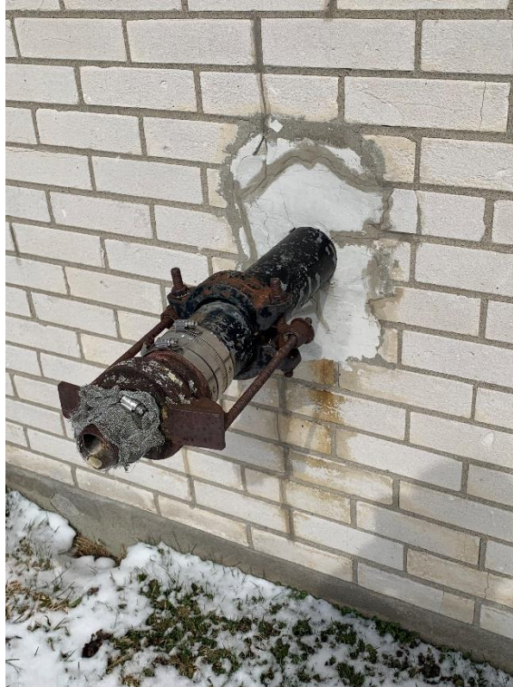
Figure A.5: Blowoff Line Protruding through South Wall of WTP
