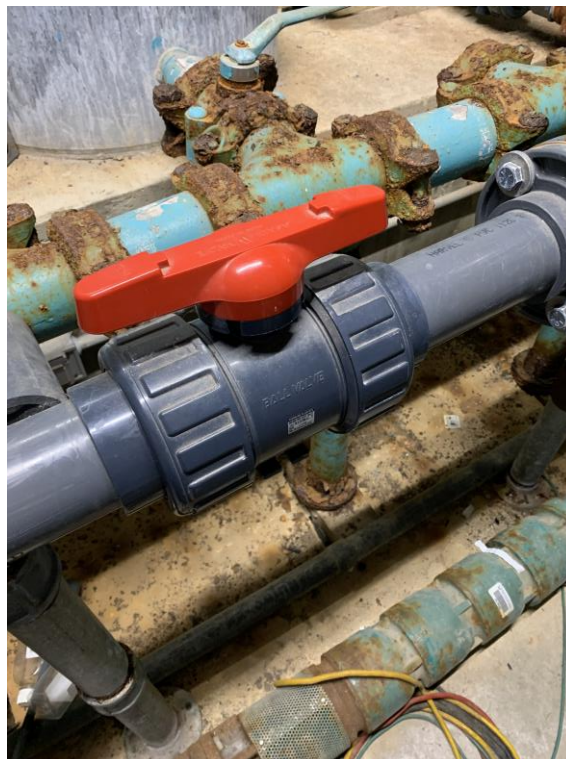
Figure A.8: Isolation Ball Valve Downstream of Flow Control Valve
