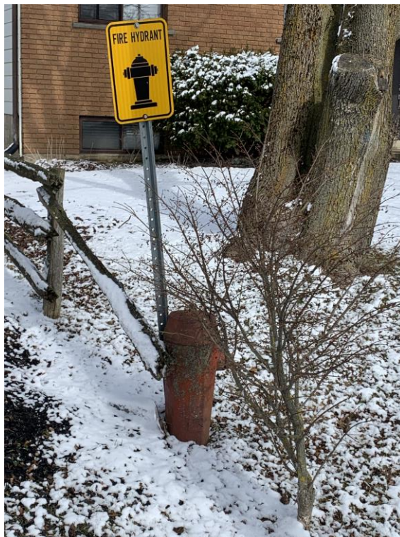
Figure A.30: Northeast Hydrant on Victoria Boulevard
