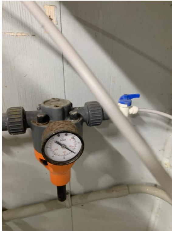
Figure A.23: Ball Valve and Backflow Preventor Upstream of Free Chlorine Analyzer
