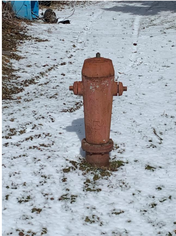
Figure A.29: Southwest Hydrant on Victoria Boulevard
