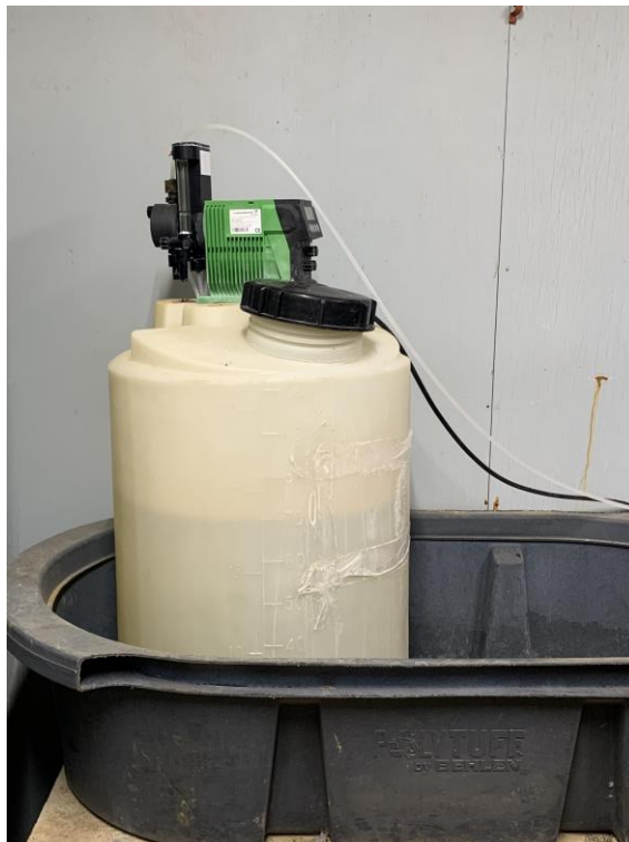
Figure A.12: Sodium Hypochlorite Storage Tank and Secondary Containment Container. The Duty Chemical Metering Pump is Located on top of the Storage Tank
