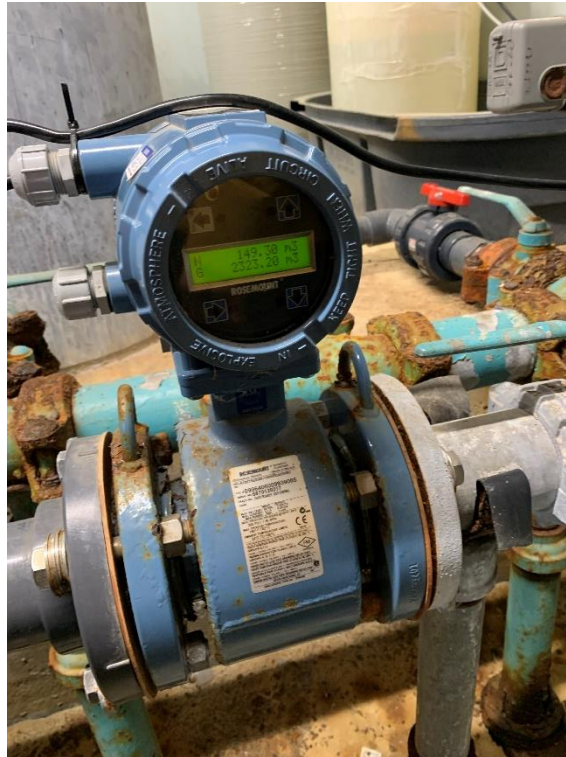
Figure A.9: Rosemount Magnetic Flow Meter
