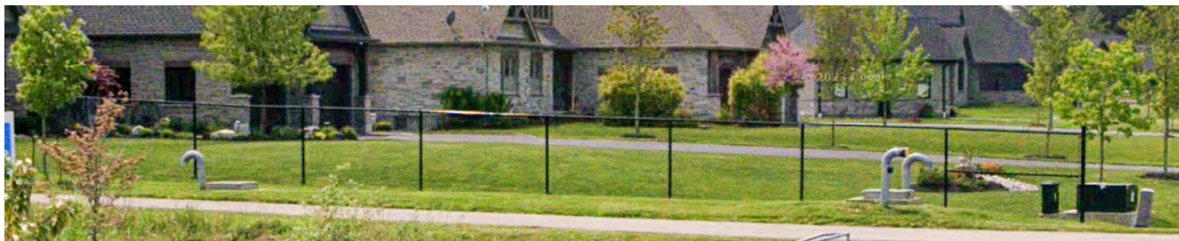
Example of an Offline Reservoir - Only vent pipes, access hatch, and draft pipe for fire department connection can be viewed above ground. Bollards are sometimes added to prevent vehicular traffic from driving/parking over the tank
